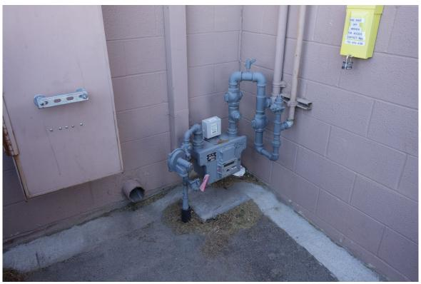
LV B&G – Public Works Office – FCA Building #0418 Description: Seismic Gas Shut-Off Valve Needed.
