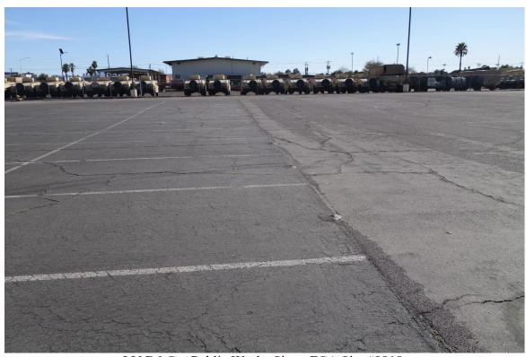
LV B&G – Public Works Site – FCA Site #9818 Description: Parking Area Crack Fill & Seal Needed.
